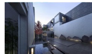
HangZhou R&D Center
